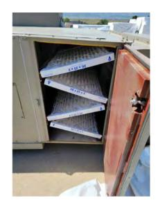
pre filter and a minimum MERV 13 final filter. If two stage filtration is not available, standalone or portable air cleaning units should come equipped with MERV 13 to HEPA filtration and be combined with UVGI for airstream disinfection. your filter supplier for proper maintenance and change out times depending on your facility.
